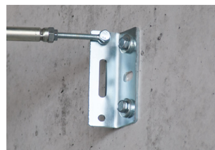
Fixing of brackets and console bearers
