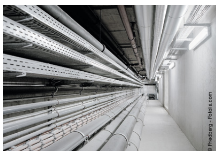
Fixing of cable ducts
